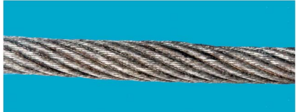
圖 113 纜徑局部增大 Local increase in rope diameter due to core distortion
